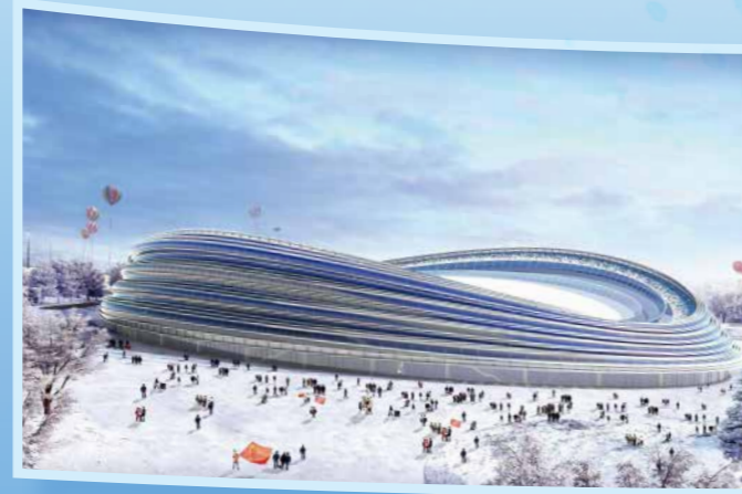
Winter Olympics - national power supply guarantee project
